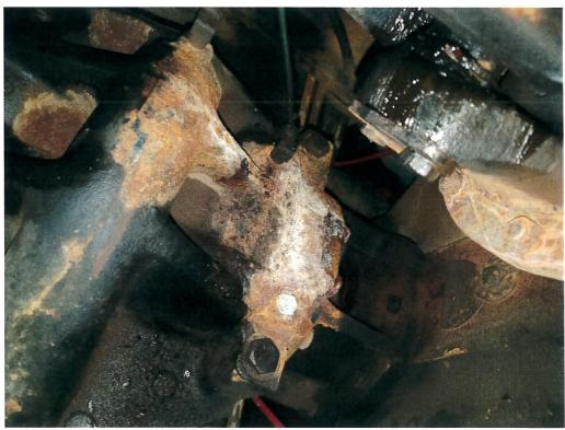
Plumbing; The plumbing is original and made from untreated steel. The plumbing shows signs of significant rust and is in need of repair/replacement at the same time the pump is repaired.
