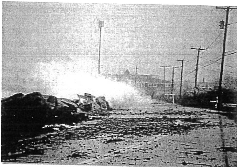
Figure 1. Storm damage on Route 1A. [Photo Credit: Kimberly Reed (1/10/13)]
