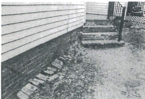
Figure 3 Apartment path and masonry stair repair
