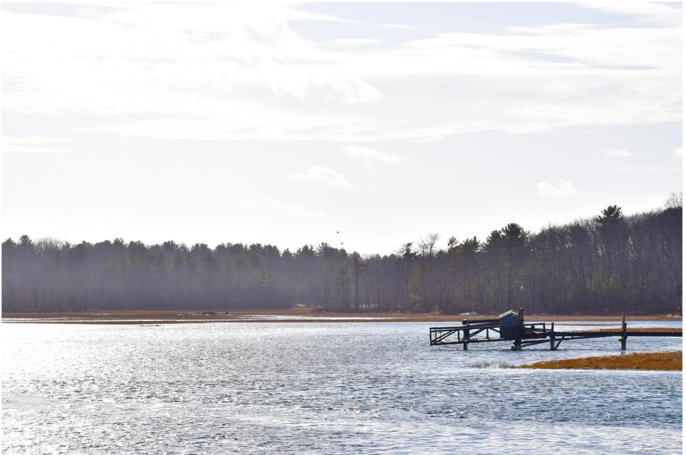
Photo #5 from bridge at Odiorne Point bridge by boat ramp:
