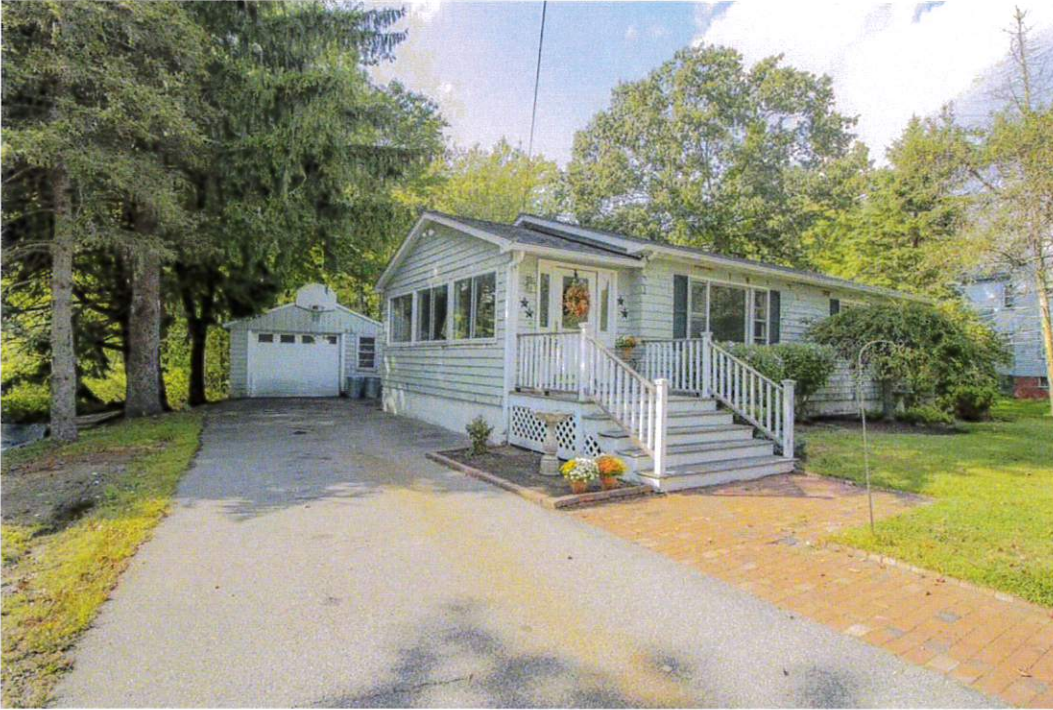
1. This is a view of the site with the trees and garage on the left side of the photo.
