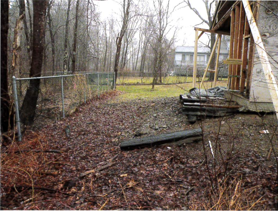
5. Looking north at the back of the garage where the shed was removed.
