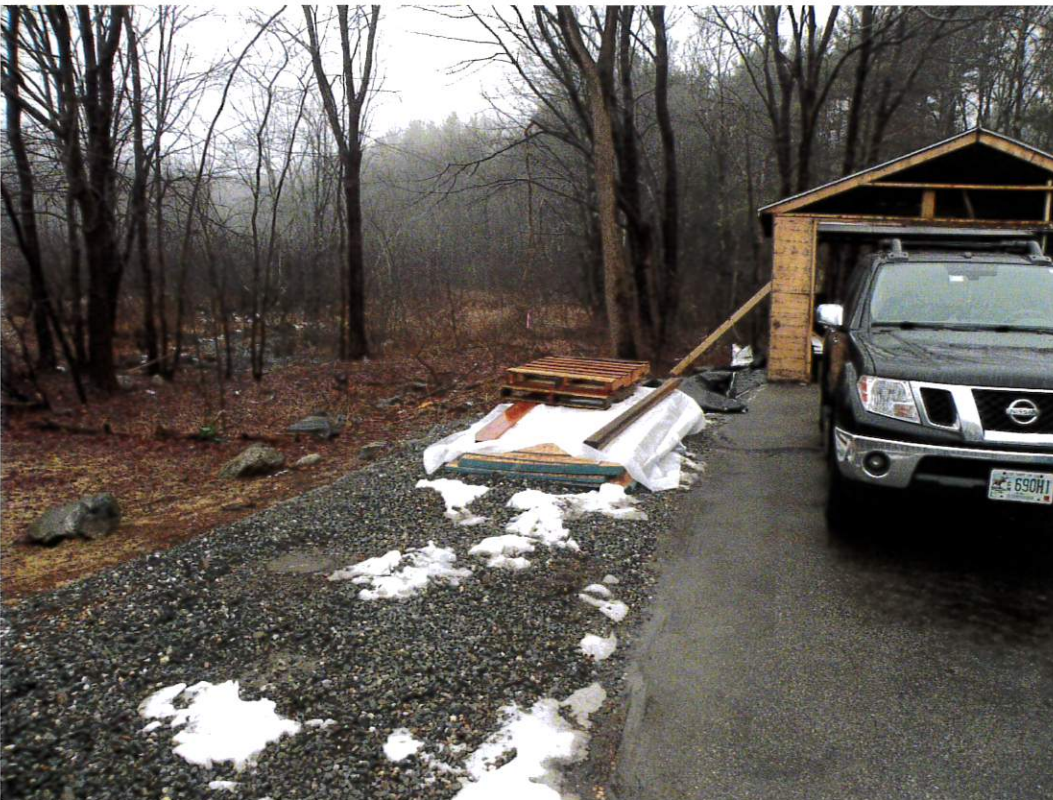
2. Looking west at the crushed stone place south of the driveway.
