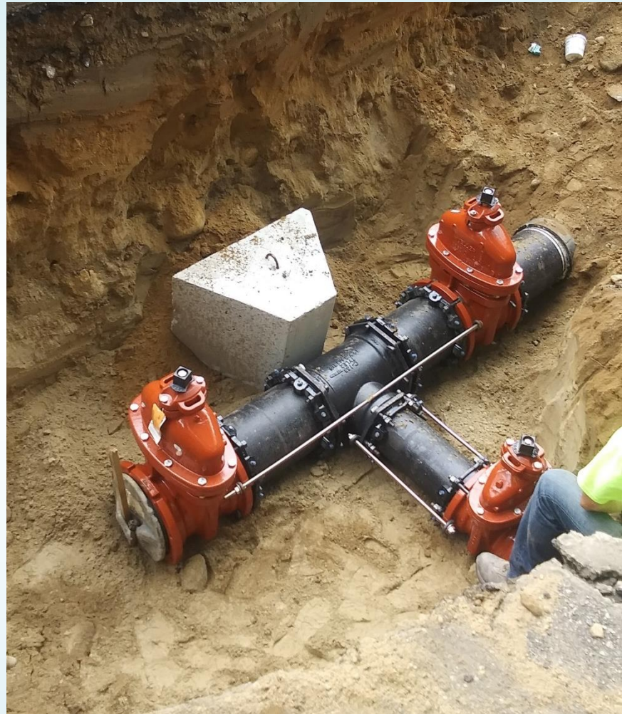
New Tee for Water Main Junction
