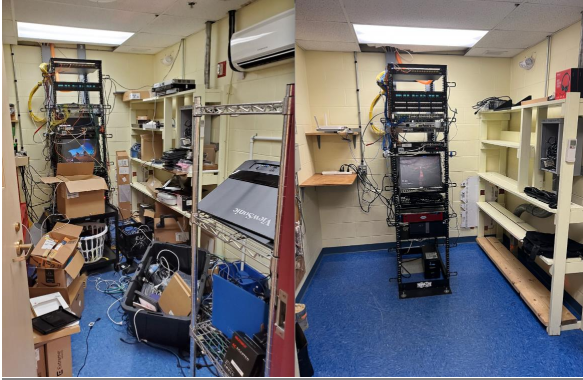
New MDF being constructed at Newington Public School:
