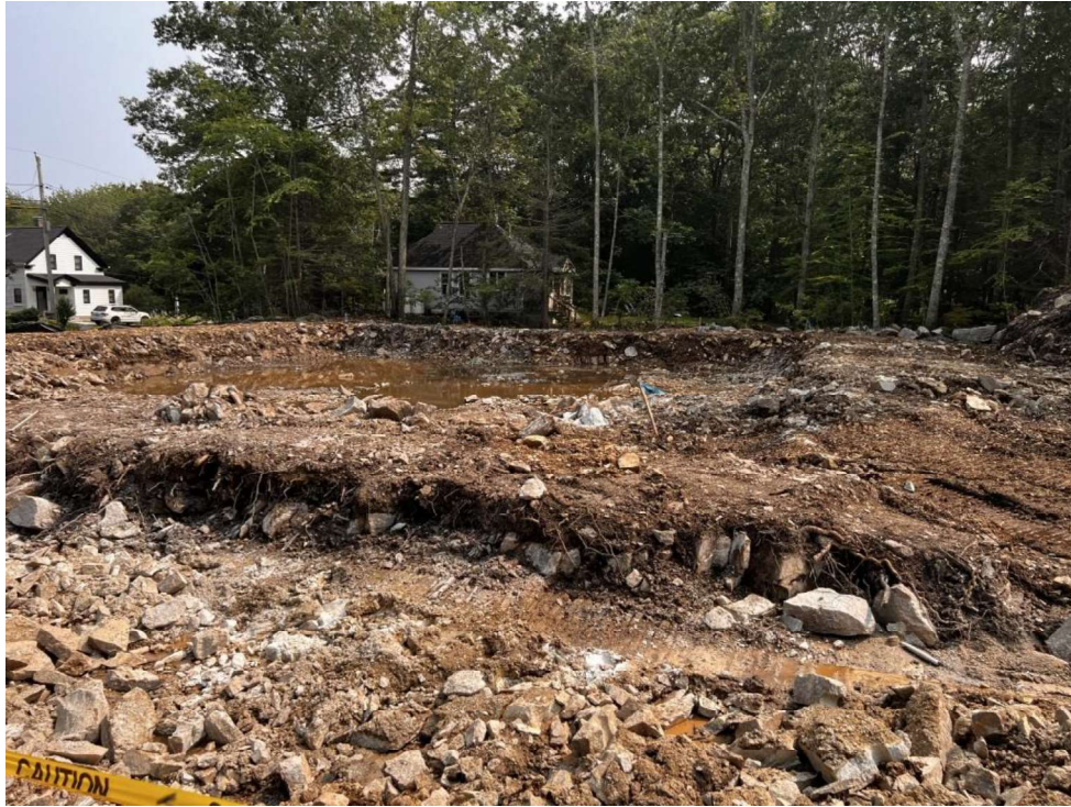
Photo 5 (07-17-23): Overall area of Bio-Retention Area #1 with blasted ledge removed.
