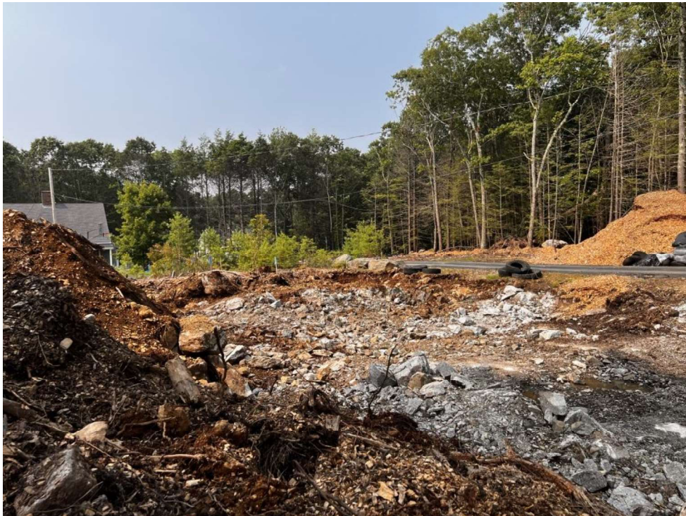
Photo 14 (07-17-23): Removal of ledge along existing driveway toward 711 Long John Road dwelling.
