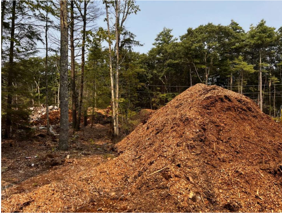
Photo 3 (07-17-23): Wood chip pile being utilized for erosion control mix berms along perimeter of site.
