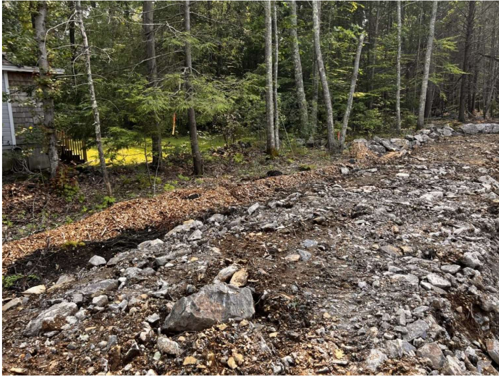
Photo 13 (07-17-23): Erosion control mix berm placed around perimeter of site and in good condition.
