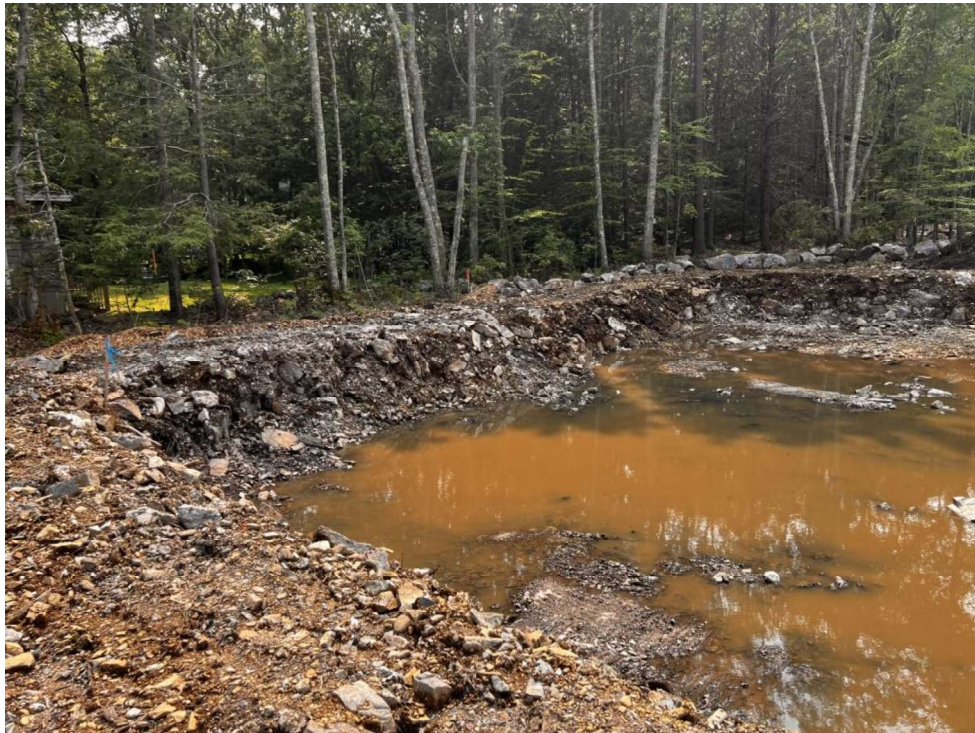
Photo 12 (07-17-23): Excavated area for Bio-Retention #1.
