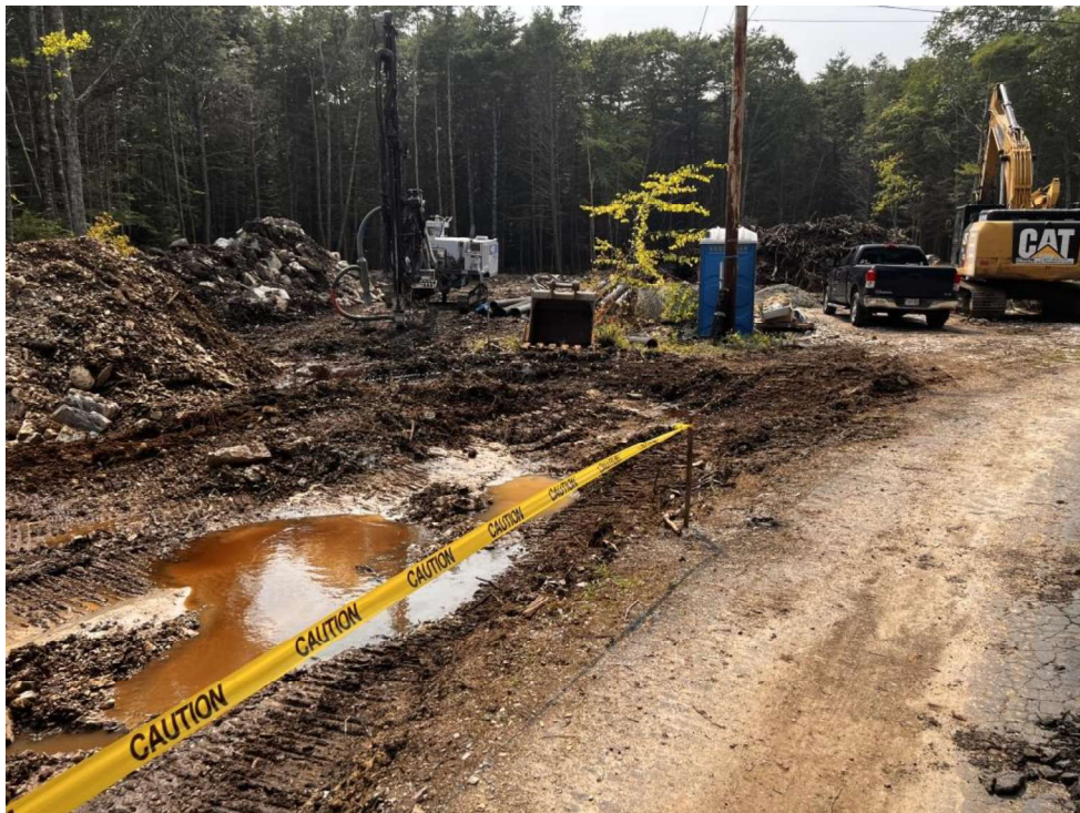
Photo 6 (07-17-23): Excavated area of sediment forebay for Bio-Retention Area #1.
