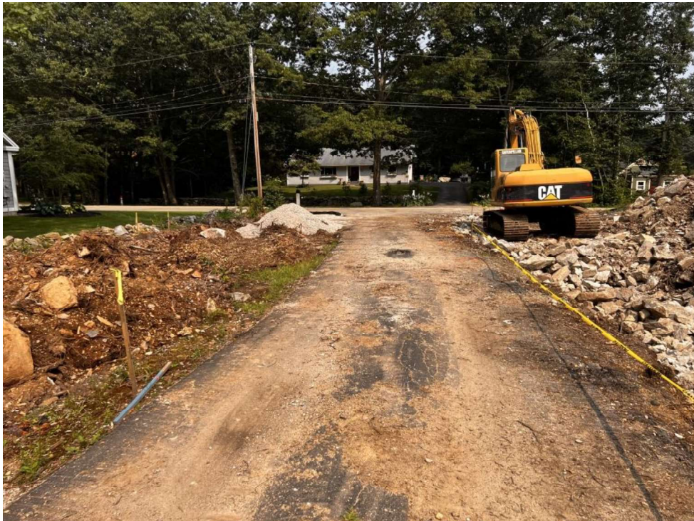
Photo 4 (07-17-23): Existing driveway facing Long John Road.
