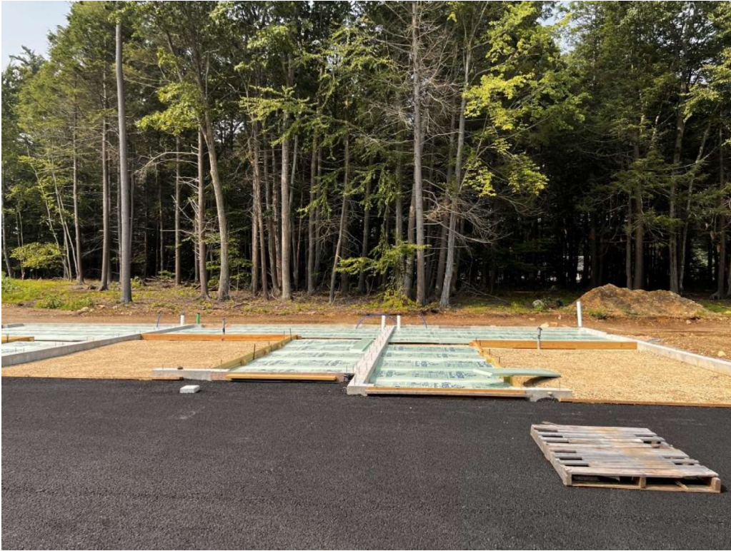
Photo 15 (07-17-23): Installation of foundation slab for Building Units 7 to 9.
