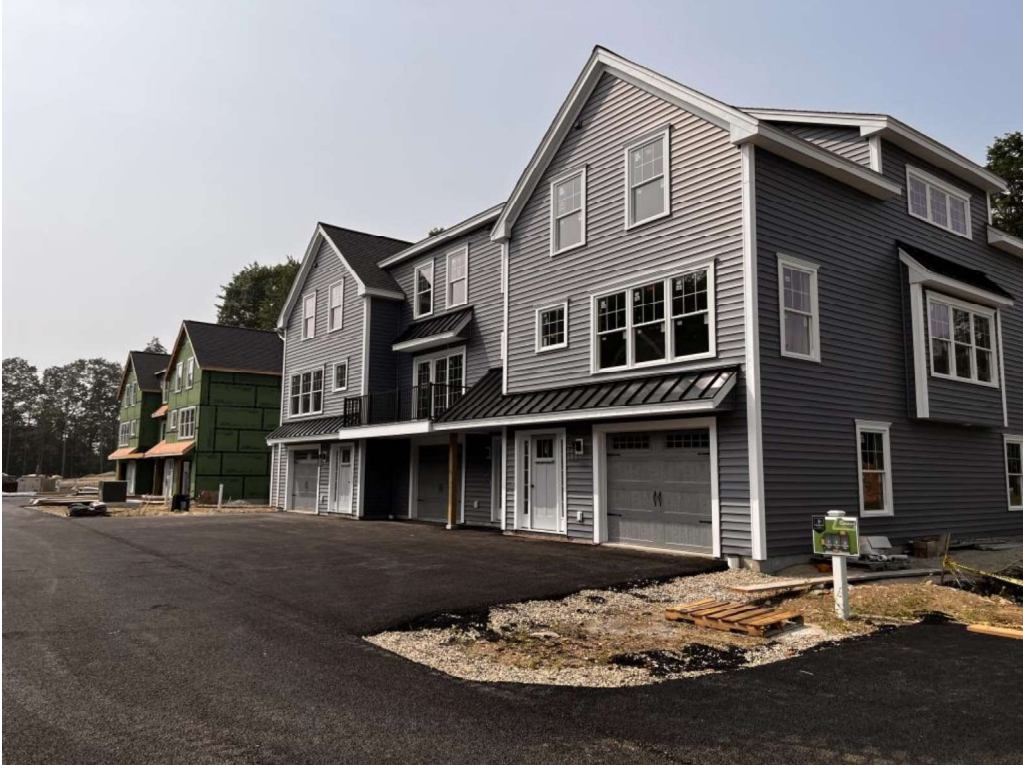
Photo 4 (07-17-23): Southeast side of Building Units 28 to 30 with exterior work complete.
