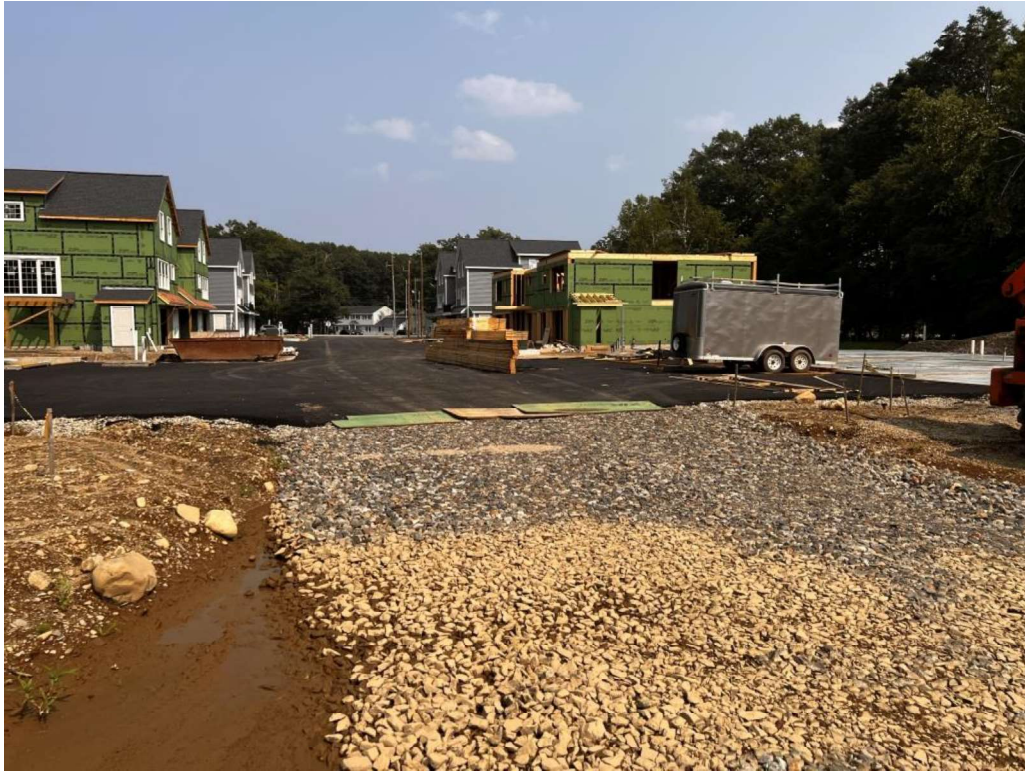
Photo 13 (07-17-23): Stabilized construction entrance on northwest end of main driveway.
