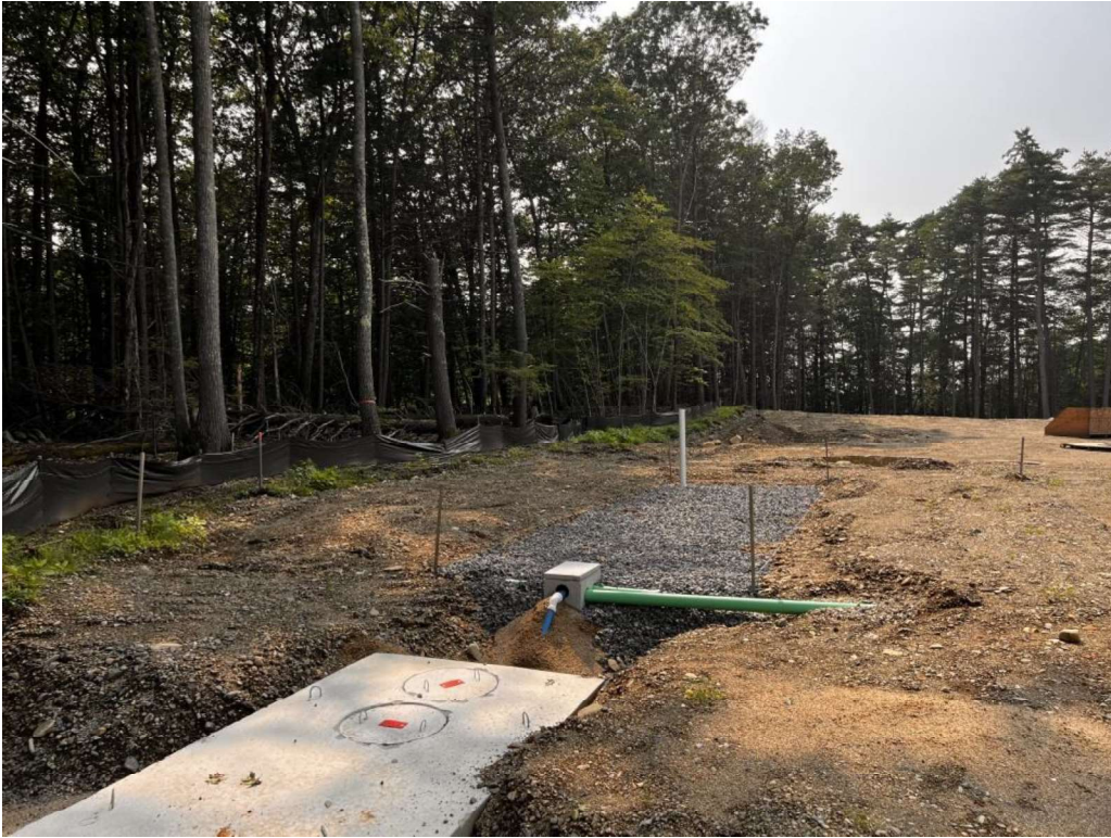
Photo 9 (07-17-23): Constructed septic system for Building Units 22 to 24.
