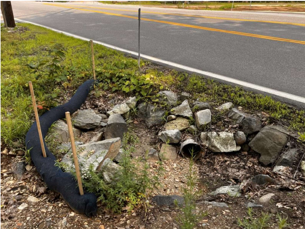
Photo 6 (07-17-23): Lafayette Road cross culvert inlet with erosion control silt sock installed.
