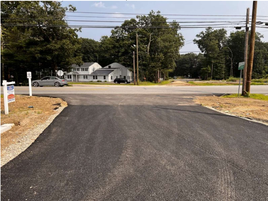
Photo 2 (07-17-23): Main site entrance facing south. No tracking observed on Lafayette Road.
