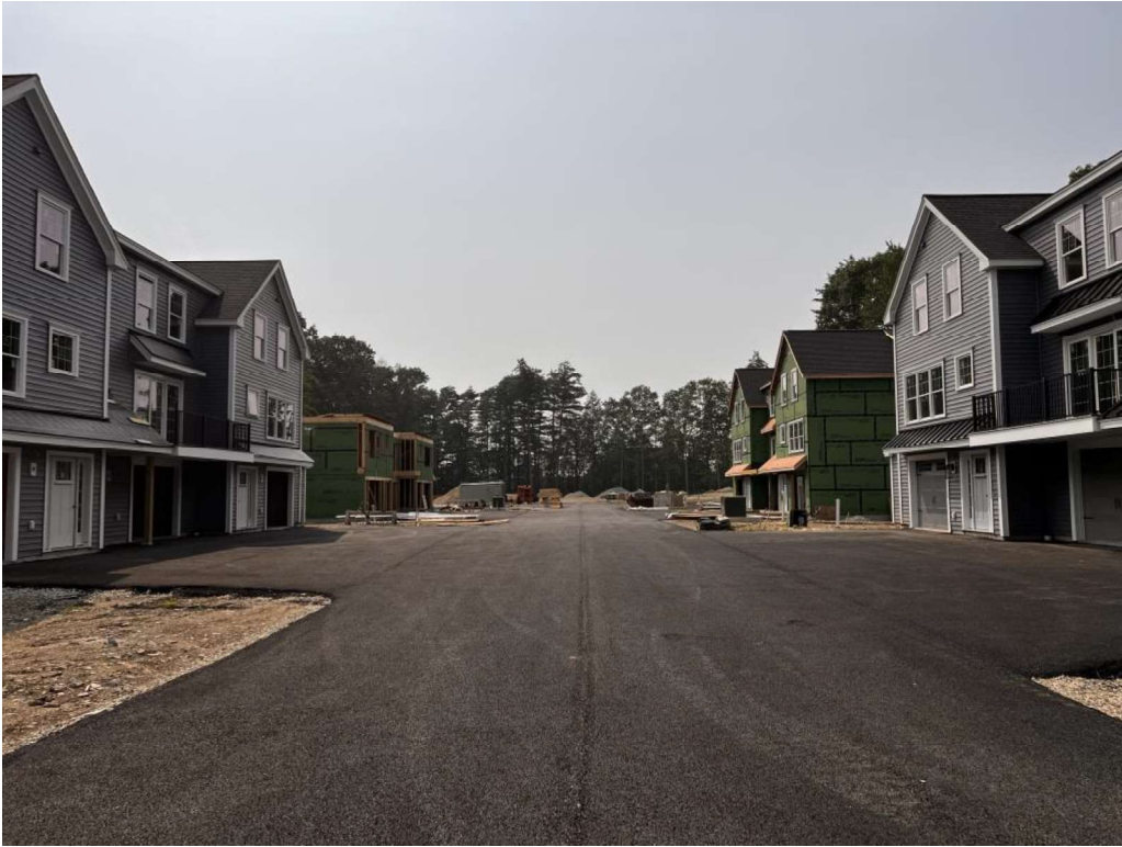
Photo 3 (07-17-23): Main driveway to site with base layer of porous asphalt.
