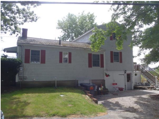
#6 464 BRACKETT ROAD (Residential)
