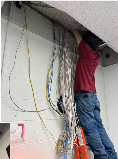
Old Wiring being pruned out
