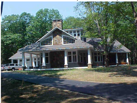
561 BRACKETT ROAD (Residential)
