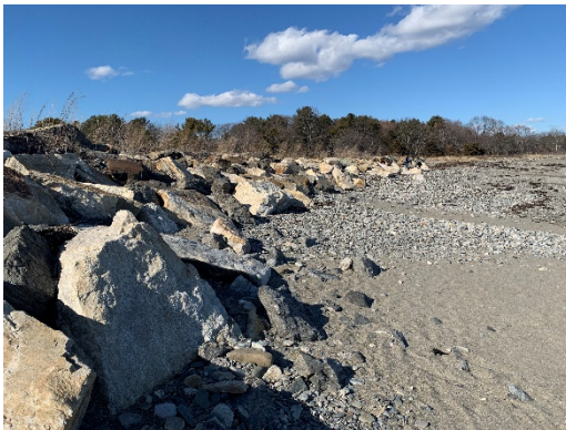
North End of Section 1 Looking Northwest
