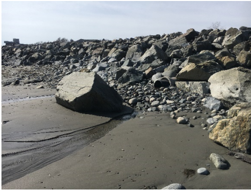
Revetment Stone Looking Southwest ( \pm Sta. 340+20)
