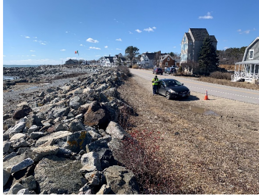
Top of Revetment Looking Southwest ( \pm End Sect.)
