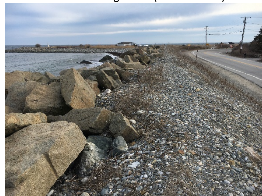
Top of Revetment Looking South Towards Begin Section 6
