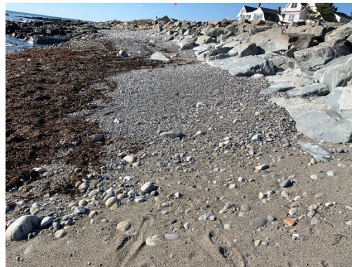
Revetment Stone Facing Looking Southwest (±Sta. 693+50)
