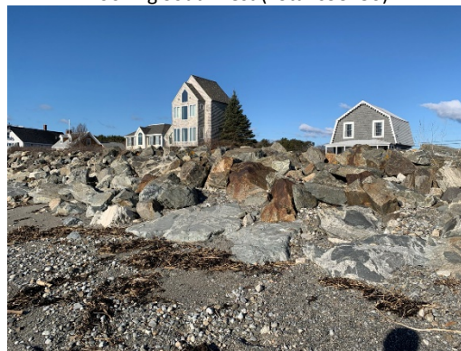
Revetment Stone Facing Looking Southwest (±Sta. 695+80)
