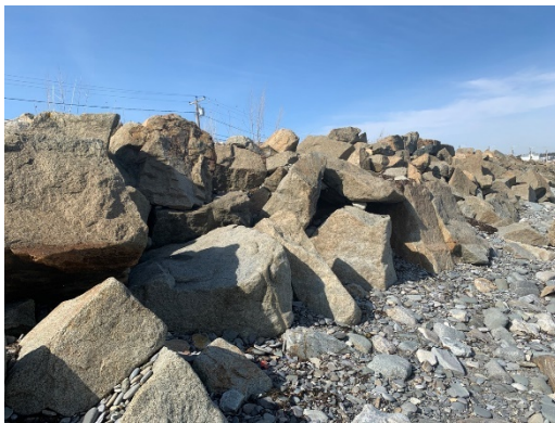
Revetment Stone Facing Looking North (±Begin Sect.)
