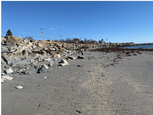
Revetment Stone Facing Looking Northeast (±Begin Sect.)
