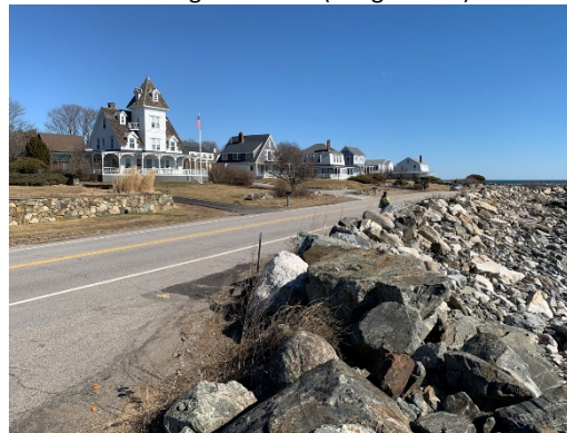
Top of Revetment Looking Northeast (±Sta 676)
