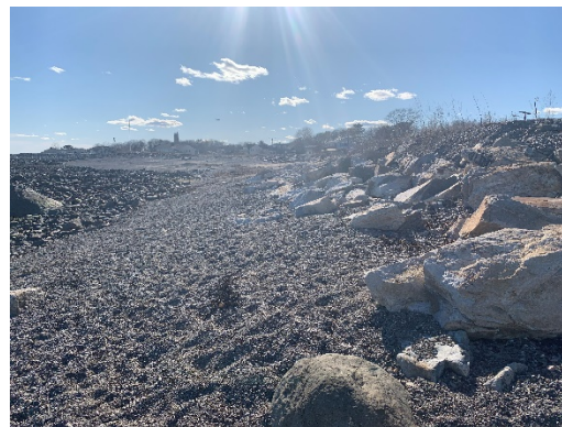
Beginning of Revetment/End of Beach Access Looking Southwest
