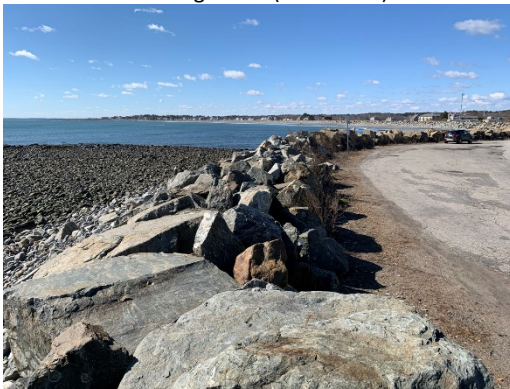
Top of Revetment Looking Southwest (±Sta 677+60)
