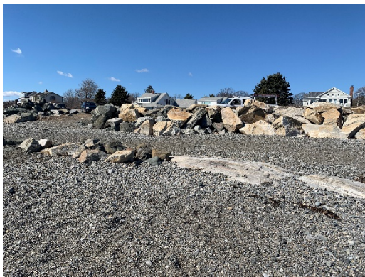
Loosely Placed Revetment Stone Facing Looking West (±Begin Sect.)
