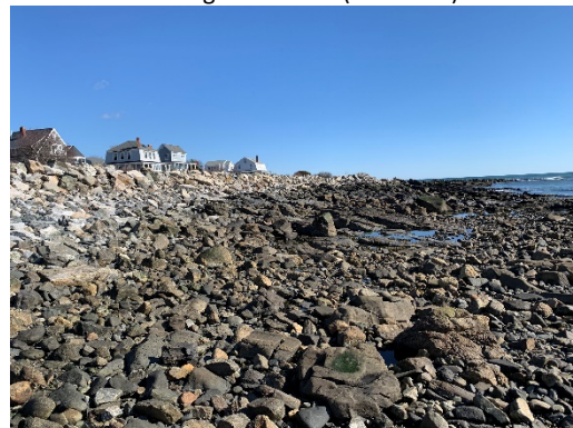
Revetment Looking Northeast
