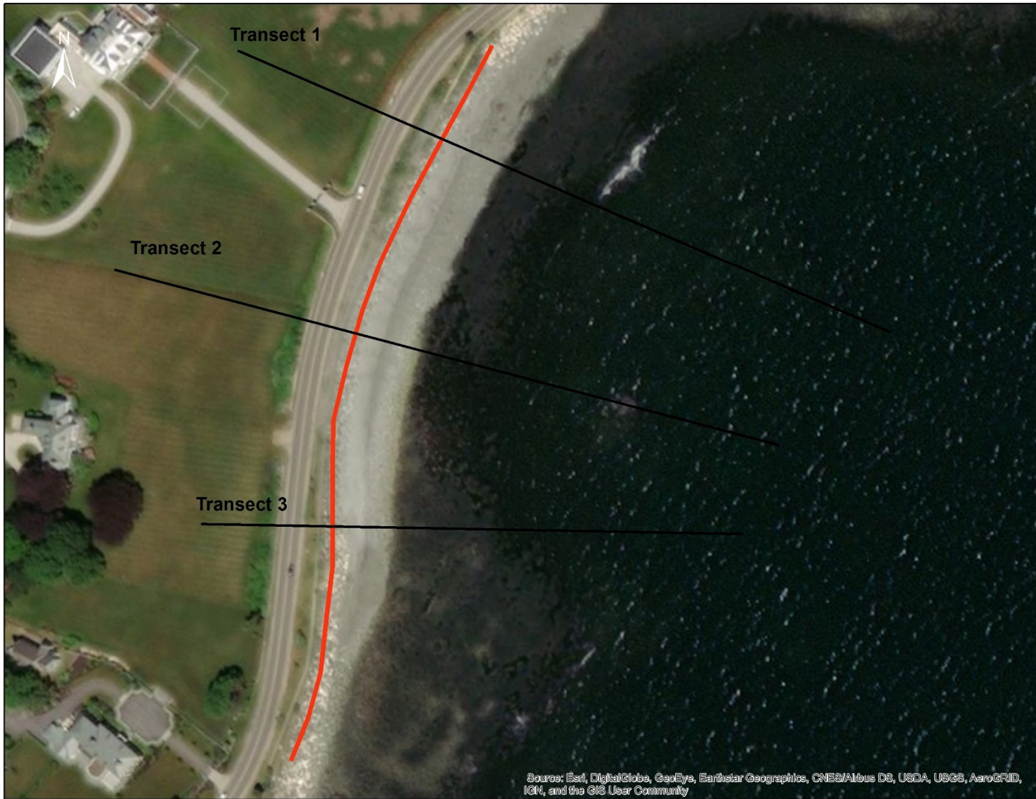
Figure 55. Transect Locations at NHDOT S.R. Section 13.
