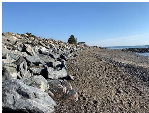
Revetment Stone Looking Northeast towards ±End Sect.
