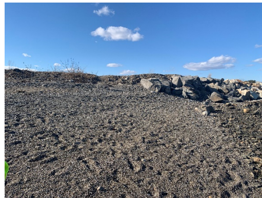
End of Revetment/Beginning of Beach Access Looking Northwest
