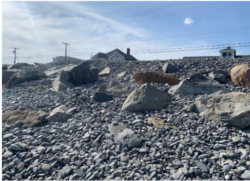
Shale Pile with Sporadic and Sparse Revetment Stone Looking Southwest (±Sta. 646)
