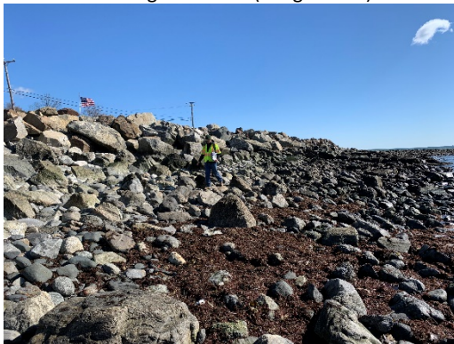
Revetment Stone Facing Looking Northeast (±Sta. 672)
