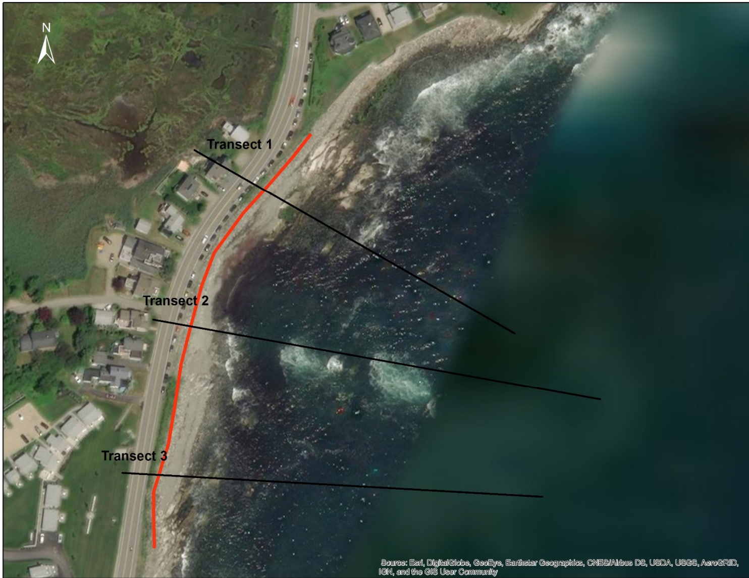
Figure 25. Transect Locations at NHDOT S.R. Section 4.
