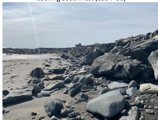
Revetment Stone Looking South
