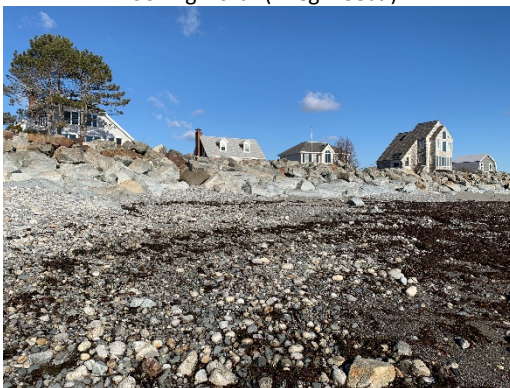
Revetment Stone Facing Looking Southwest (±Sta. 694)
