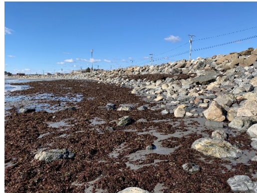
Revetment Stone Facing Looking Southwest
