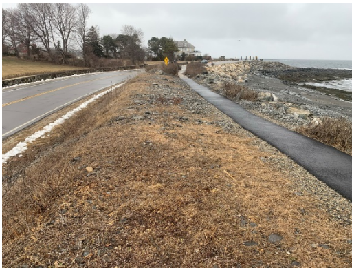
Top of Revetment Defined Walking Path Looking North ( \pm Sta. 280+30)
