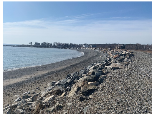
Top of Revetment Looking Southwest
