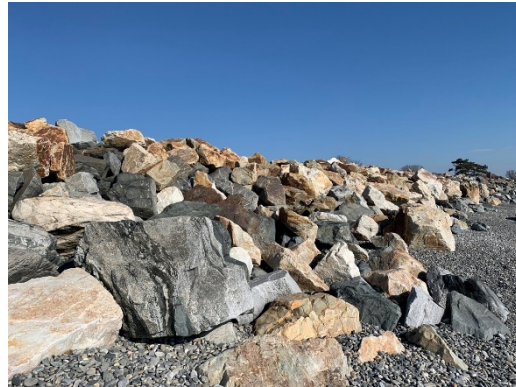
Revetment Stone Looking North (±Sta. 304+60)
