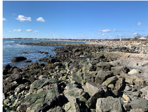
Typical Revetment Looking Southwest (±Sta. 677 – Sta. 680+50)
