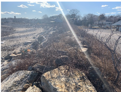
Top of Revetment Looking Southwest
