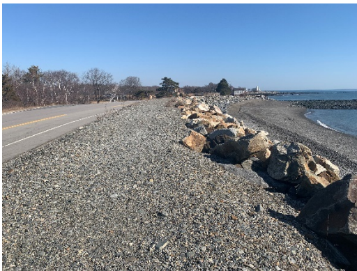
Top of Revetment Looking North towards ±End Sect
