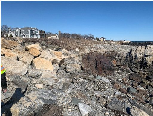
End Revetment/Beginning Beach Access & Shale Pile Looking Northeast ( \pm Sta. 773)
