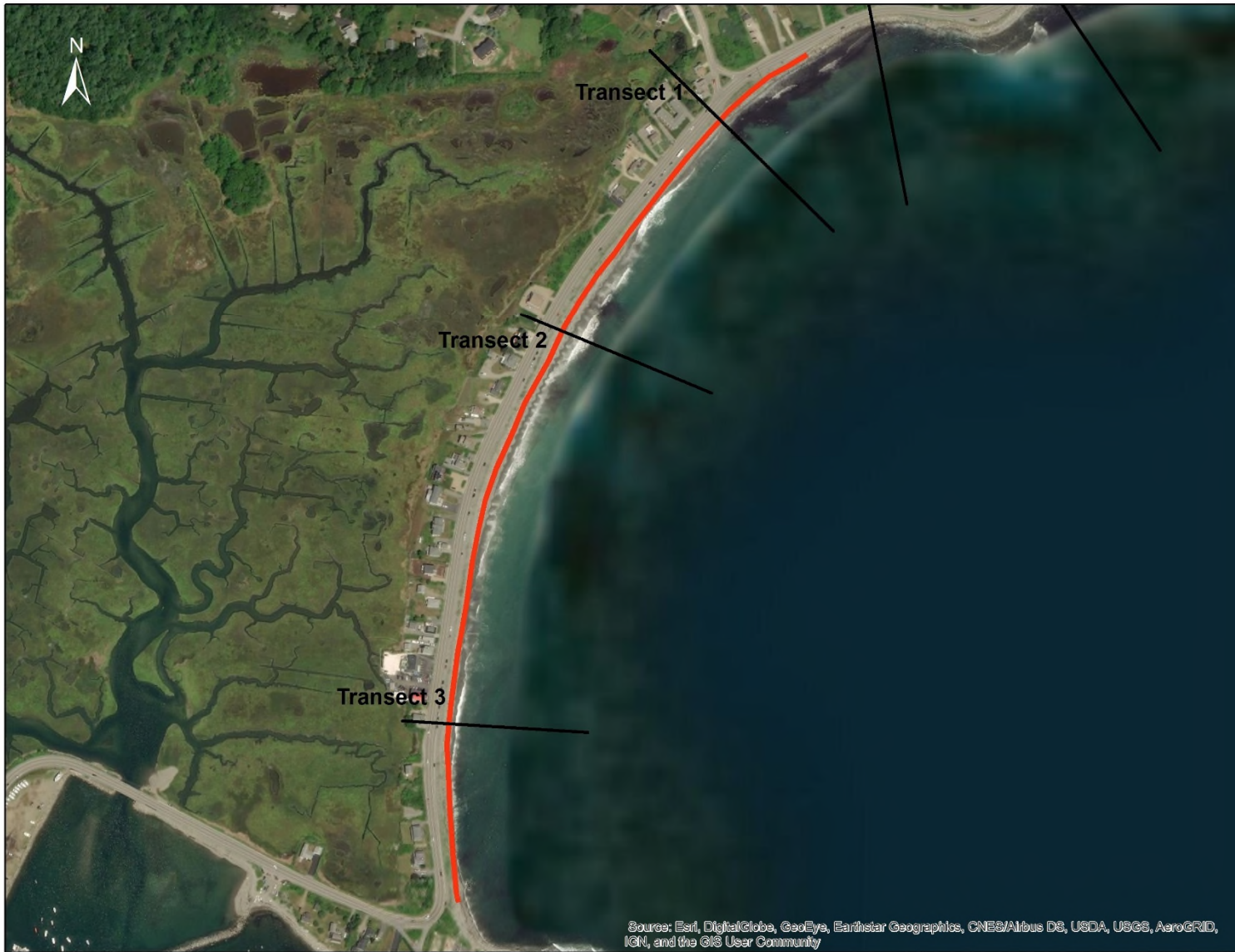
Figure 37. Transect Locations at NHDOT S.R. Section 6.
