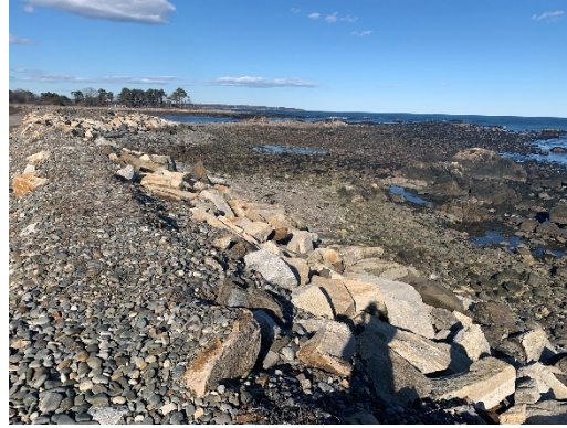
Top of Revetment Looking Northeast (±Begin Sect.)
