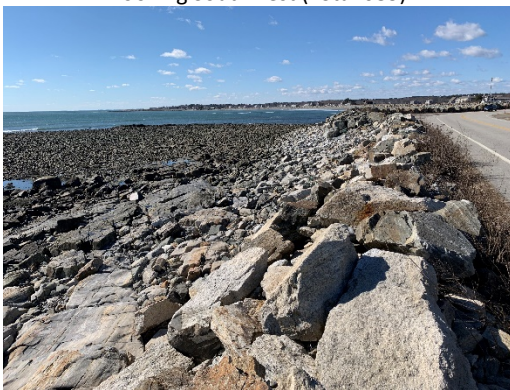
Top of Revetment Looking South (±End Sect.)
