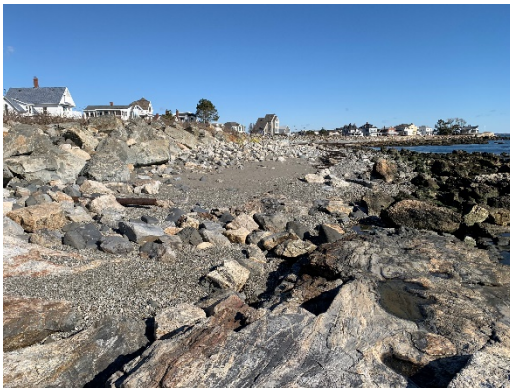
Revetment Stone Facing & Beach Bench Looking North (±Begin Sect.)
