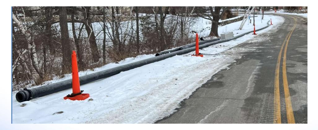
Installed 300 feet of new High Density Polyethylene (HDPE) water main and a valve
