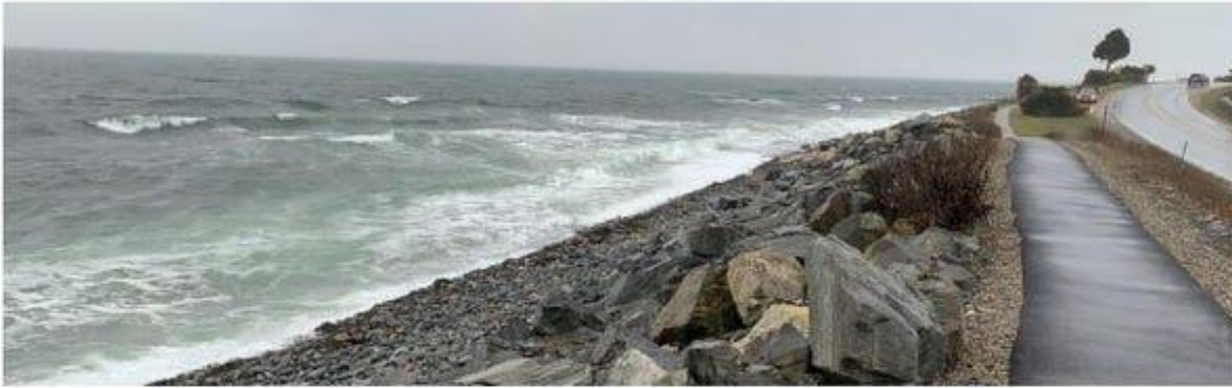
Figure 1: NH Rt 1A, Section 13 – Revetment with pedestrian path
