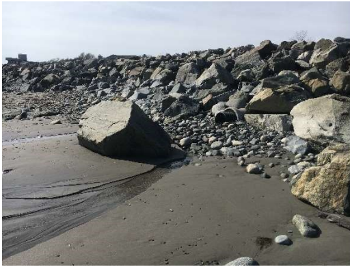
Revetment Stone Looking Southwest ( \pm Sta. 340+20)
