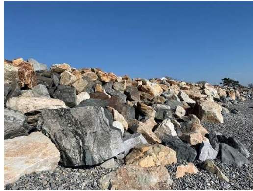
Revetment Stone Looking North (±Sta. 304+60)
