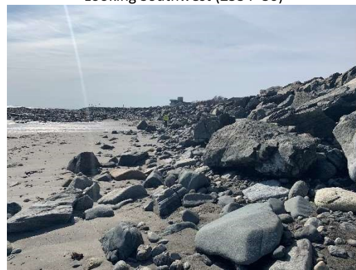
Revetment Stone Looking South
