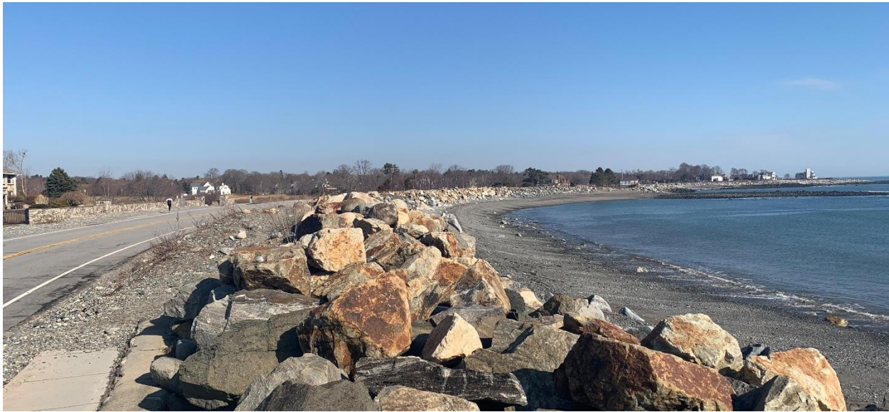
Figure 10: Revetment stone on NH Rt 1A
