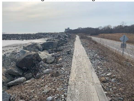
Top of Revetment; Defined Walking Path Looking Southwest ( \pm 344+40)
