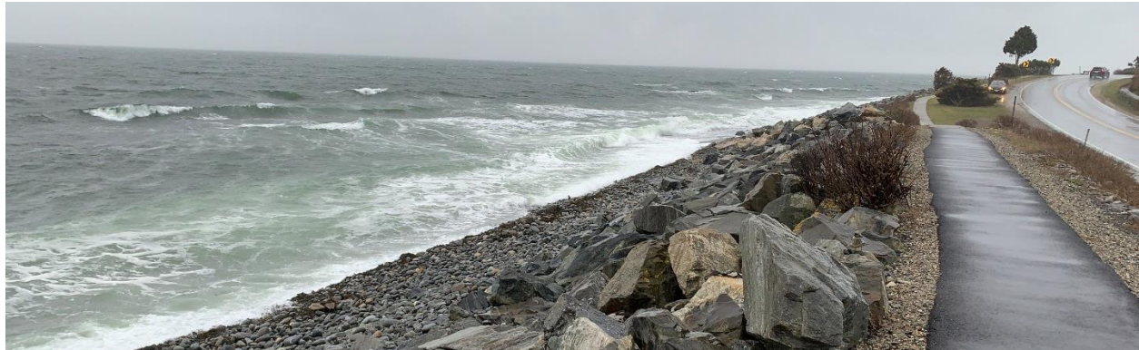
Figure 1: NH Rt 1A, Section 13 – Revetment with pedestrian path
