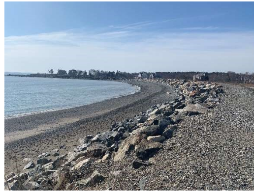
Top of Revetment Looking Southwest
