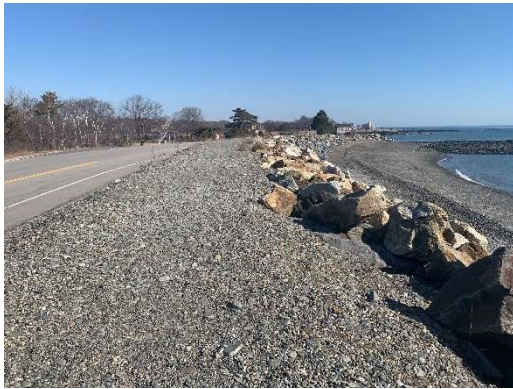
Top of Revetment Looking North towards ±End Sect
