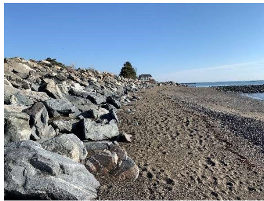
Revetment Stone Looking Northeast towards ±End Sect.
