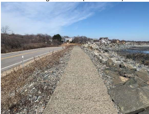
Top of Revetment; Defined Walking Path Looking Northwest ( \pm Begin Sect.)
