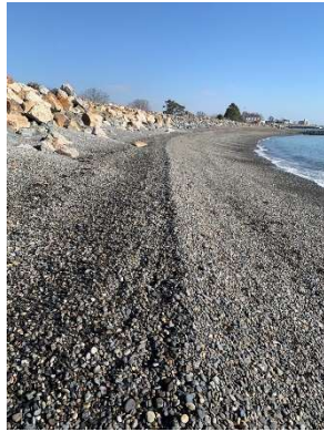
Revetment Stone and Cobble Berm Looking Northeast (±Sta. 303)
