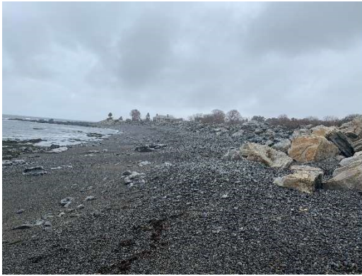
Revetment Stone Looking South ( \pm End Sect.)
