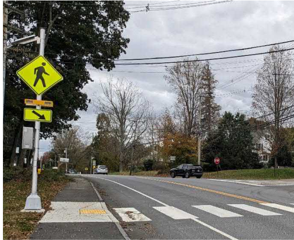
RECTANGULAR RAPID FLASHING BEACON
