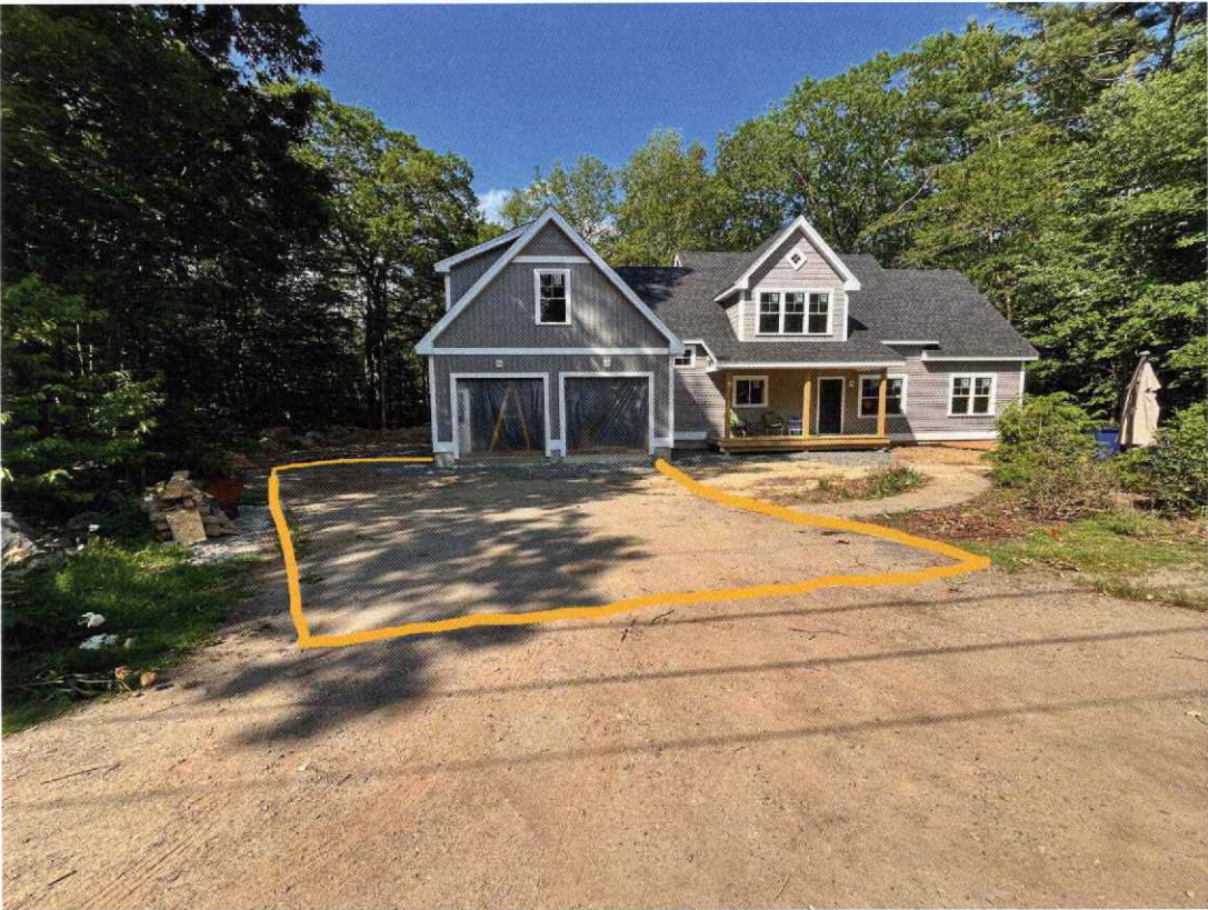
15 Vinmar Court, driveway application
