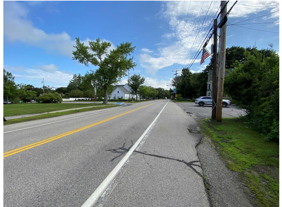
Approaching Olde Parish Road Looking North
